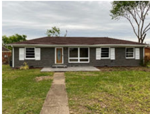
Property after repairs
